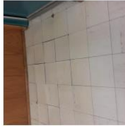
CES replace floor in multipurpose room
