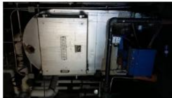
CPS Install new boiler - CT
