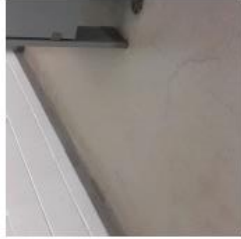
AES Replace Epoxy bathroom floors
