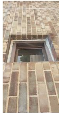
CHS Replace Library Windows CT
