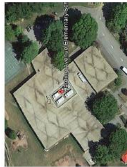
HAE HVAC Units Replacement?
